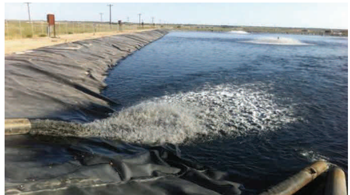
Discharge of recovered water to a centralised pit for reuse
