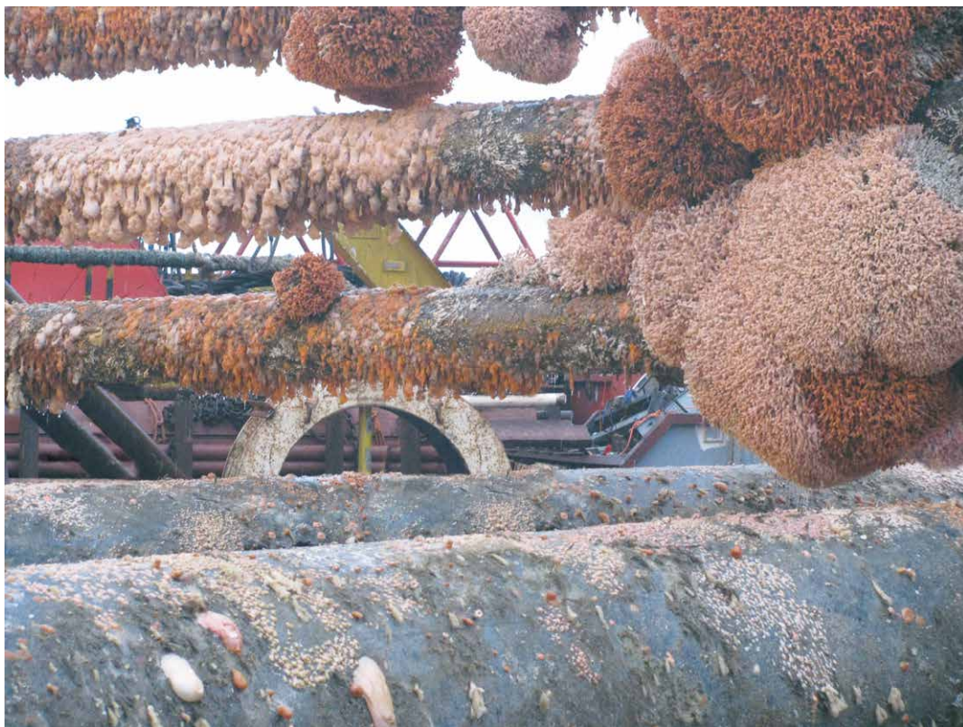
Figure 7: The ability of the marine environment to adapt to installations is evident from this cross brace removed during decommissioning of the small steel jacket platform (Photo: Heerema) .
