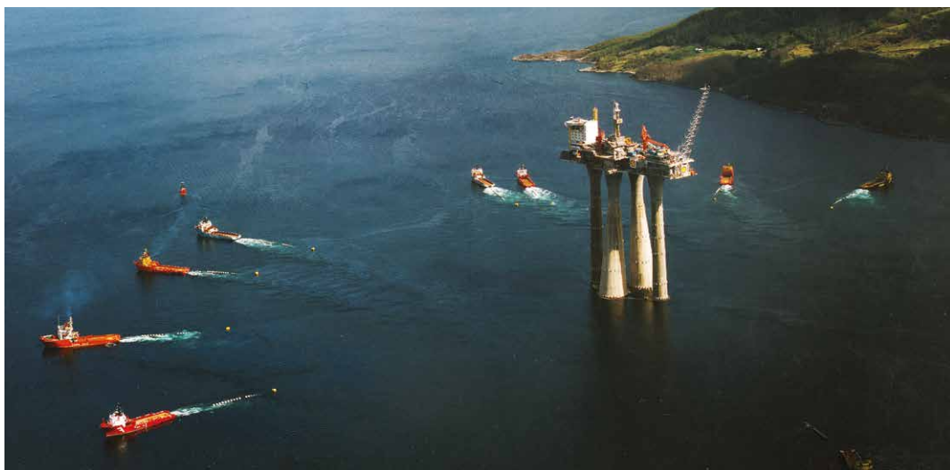
Figure 2.3: The tow-out of the Troll A CGBS – two thirds of the structure is underwater
