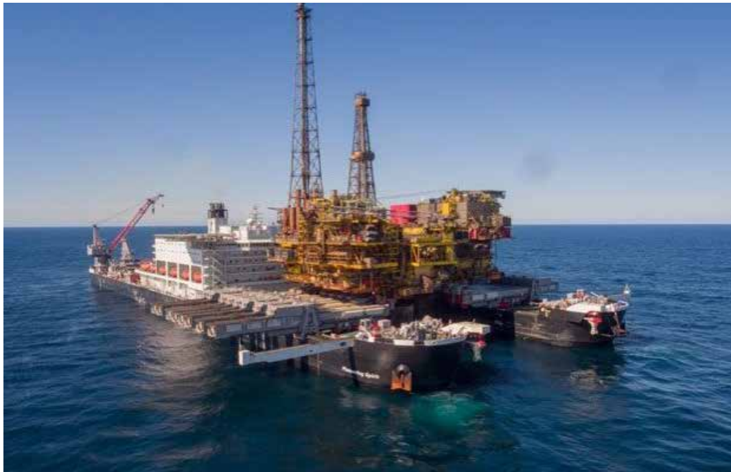
Figure 6: Brent Delta during removal of its 23,500 tonne topsides from the GBS by Allseas “Pioneering Spirit” single lift vessel
