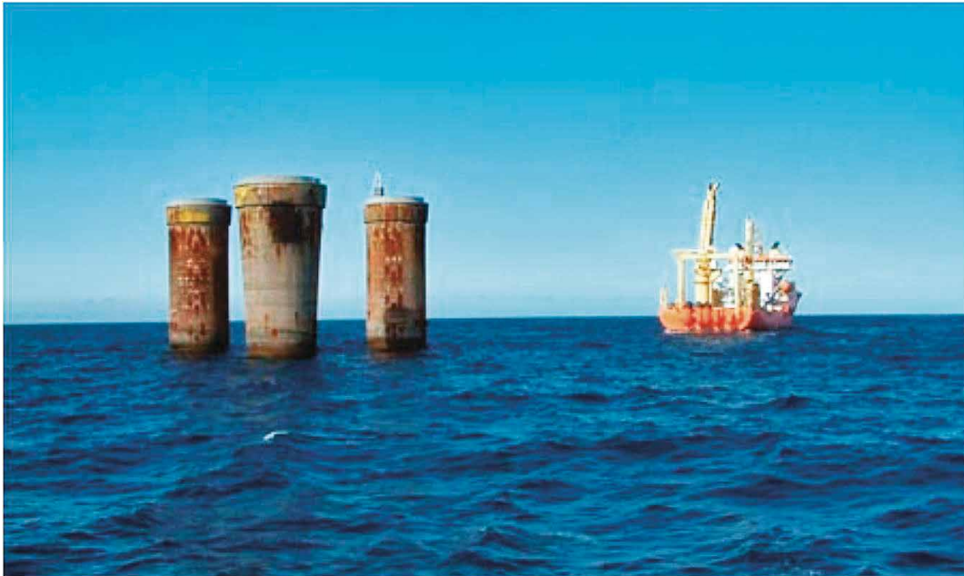
Figure 5.6: The remains of a decommissioned CGBS in the Frigg field (Photo: Saipem) .
