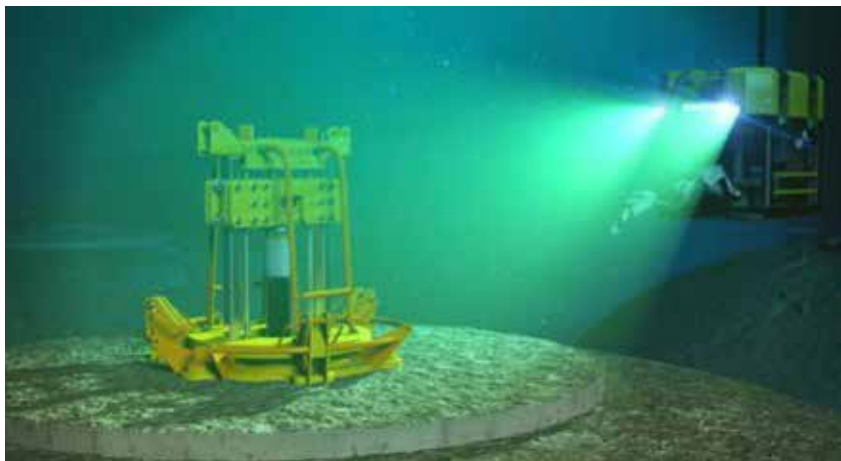
Figure 7.8.3: ROV operated equipment located on the top of GBS cell to drill and deploy survey equipment (Photo: Enpro Subsea Ltd).
