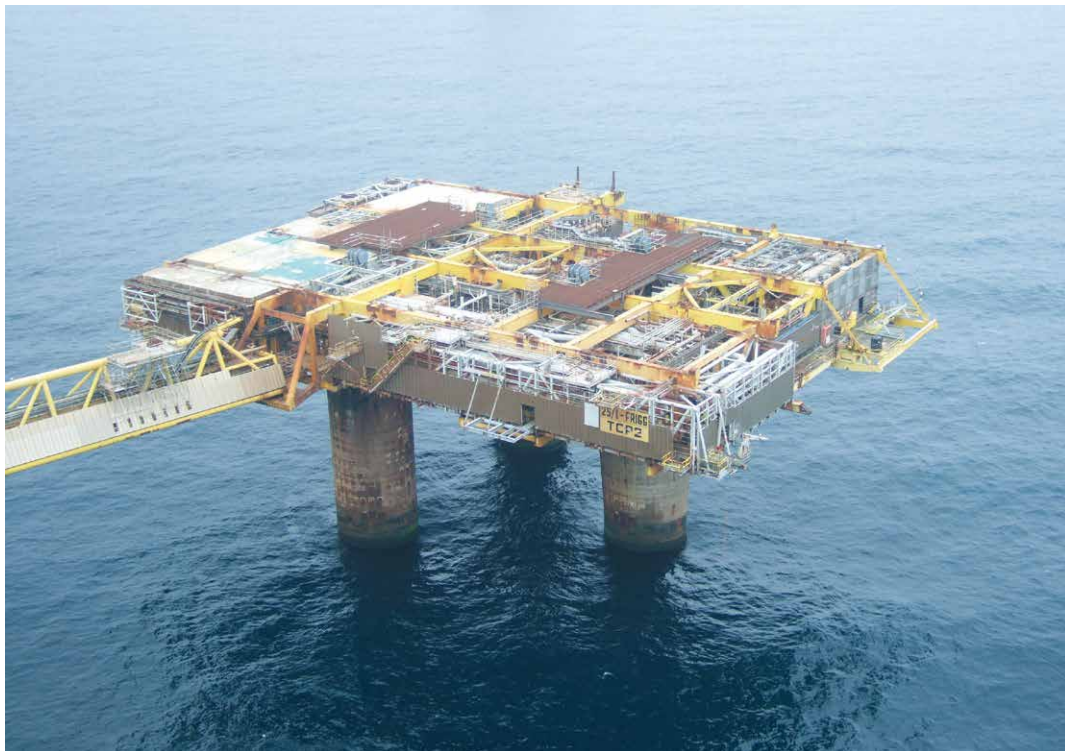
Figure 8.2: TCP2 being prepared for removal of the module support frame by a heavy lift vessel (Photo: Total).
