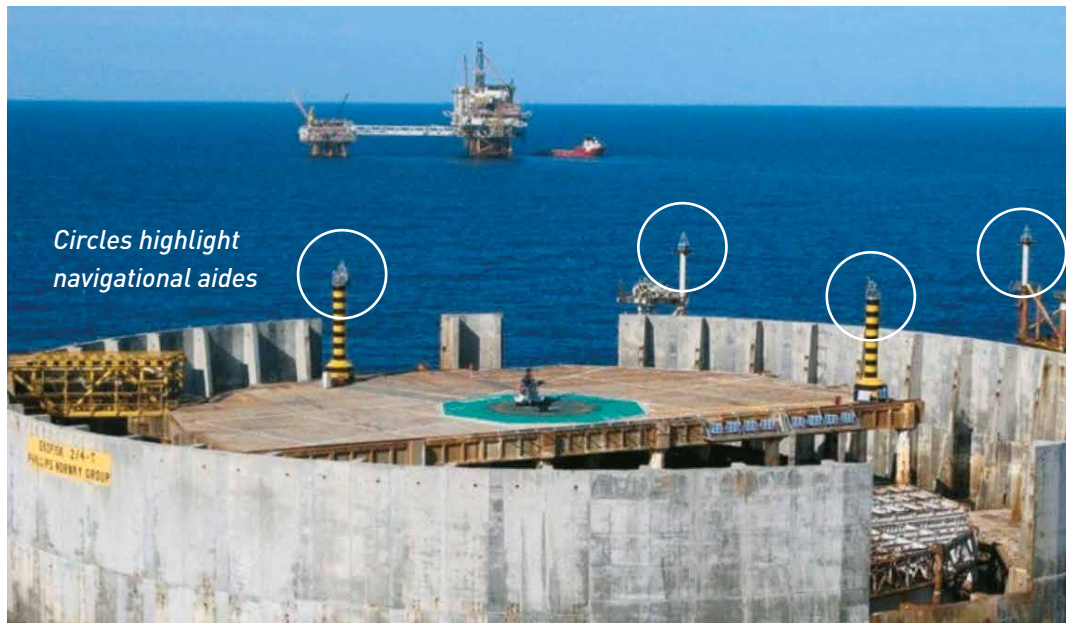
Figure 9.1: Long service interval navigational aids on the decommissioned Ekofisk Tank (Photo: ComPower/ConocoPhillips)
