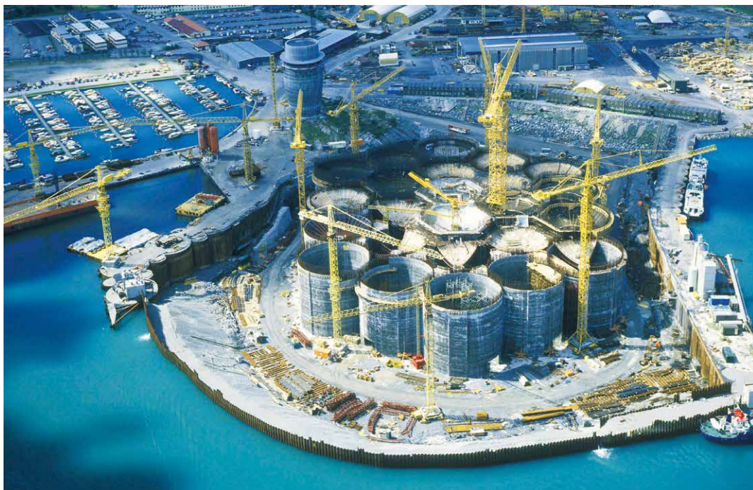
Figure 5.3: Gullfaks A under construction in a dry dock (Photo: Leif Berge / Statoil).
